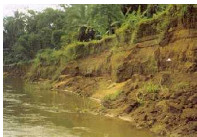
Figure 3: Exposed bank of a river due to unrestricted mining activities
